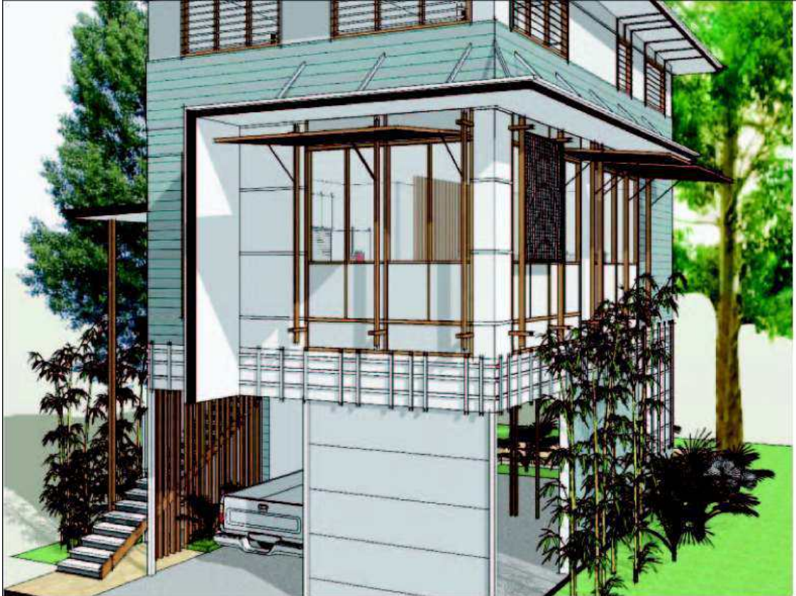
Award winning: A Brisbane architect's flood-safe design allows the water to flow through the building without placing pressure on the structure
